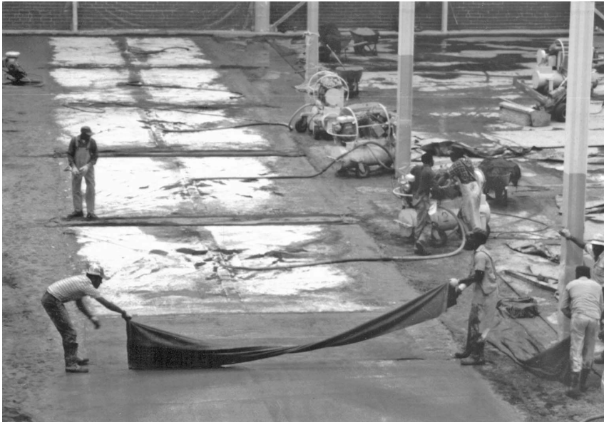
FIGURE 15.5 Distribution of vacuum pads on newly placed concrete slab.
